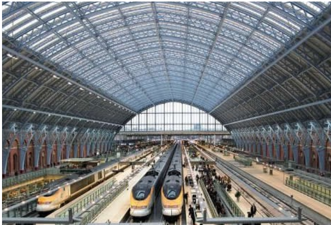
St. Pancras International Station
